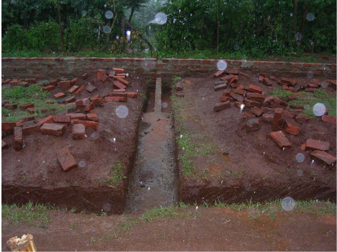
Under construction, the secondary school wing
